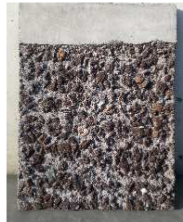
Fig.7 Façade surface texture.
