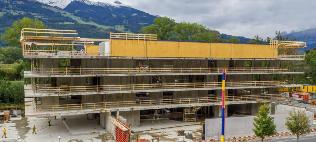
Fig. 4: Side view of building “Belvedere” at end of structural work
