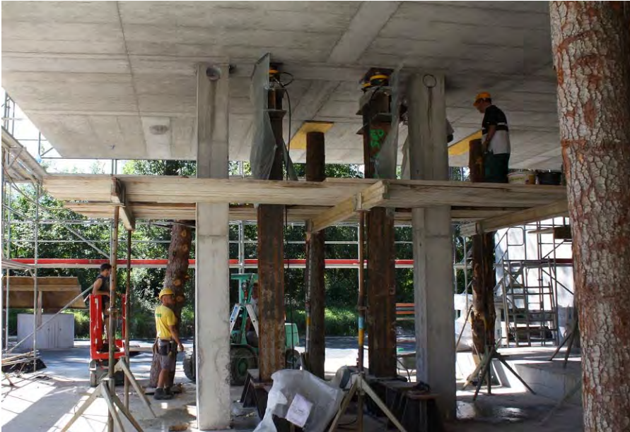
Fig. 10: Demolition of temporary concrete columns
